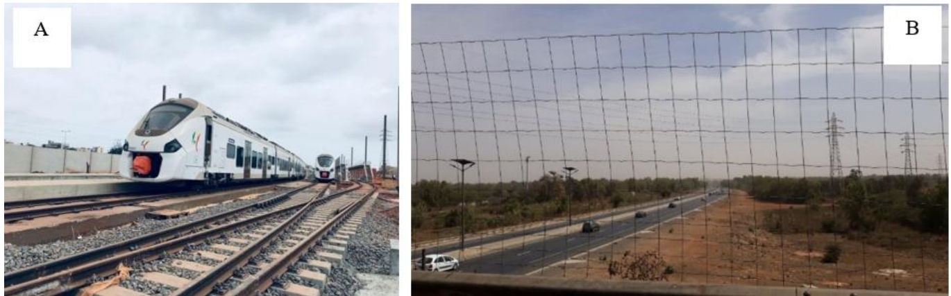
Photo 5 A, 5B : ligne ferroviaire et Train Express Régional / railway line and the regional express train (A) ; autoroute à péage qui fragmente la FCM/ toll highway that fragments the classified forest of Mbao (B)
